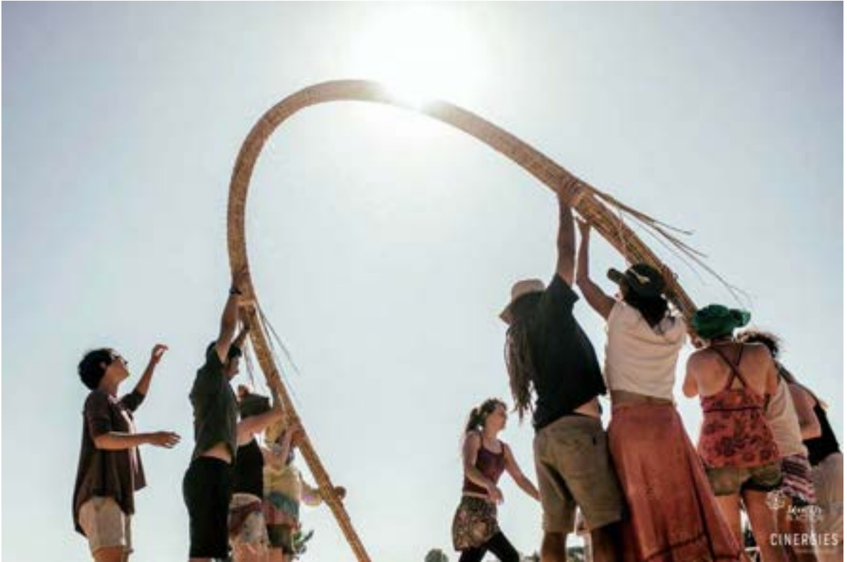
17. Building a shade structure using natural building techniques
